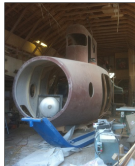
Sub building in process
